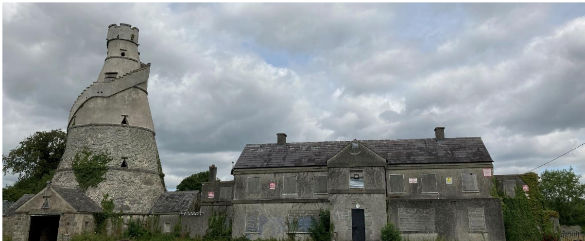
Figure 3-3: The Wonderful Barn and Existing Outbuildings
